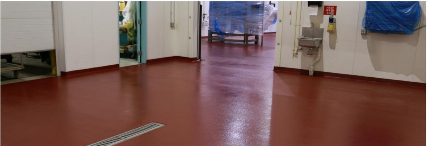
**Grease & Other Contaminants:** Exposure to grease introduces a host of issues for any food & beverage environment. It is important that any flooring system have the capability to stand up against grease contamination as well as the cleaning protocols in place to remove grease on a daily basis.
