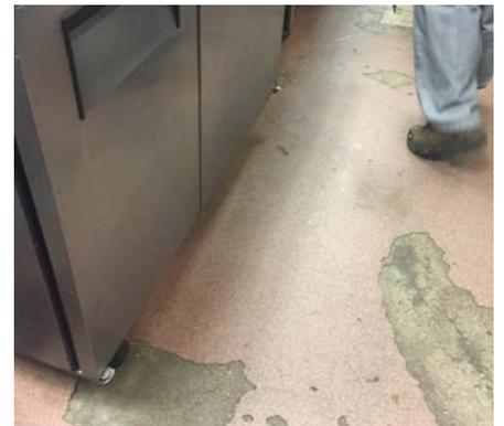
once contaminated the cracks began to delaminate and lead to flooring failure
