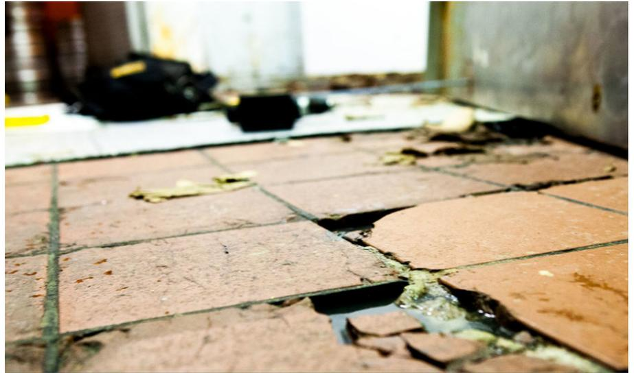
persistant expansion and contraction resulting thermal shock can cause tile grouts to fail and seperate
