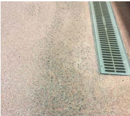
hot water exposure severely damaged this existing epoxy coating
