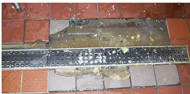
voids or pockets in a flooring system that collect water can harbor bacteria and cause severe flooring issues
