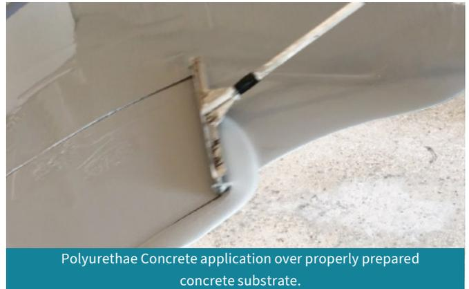
Polyurethane Concrete application over properly prepared concrete substrate.
