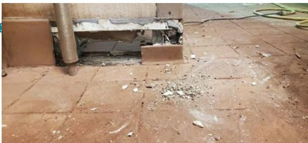
grease and contaminant build-up can lead to tile grout failures and eventual delamination
